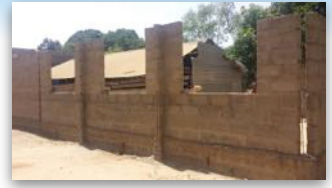
Church before roof.
