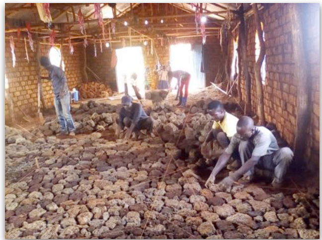
Workers laying stones for the floor.
