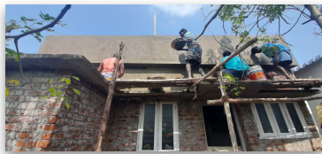
The final coat of plaster being applied to the Shriviliputher Church!
