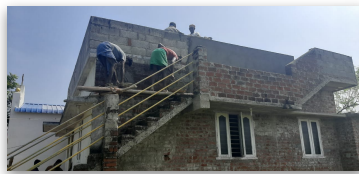
The final coat of plaster being applied to the Shriviliputher Church!
